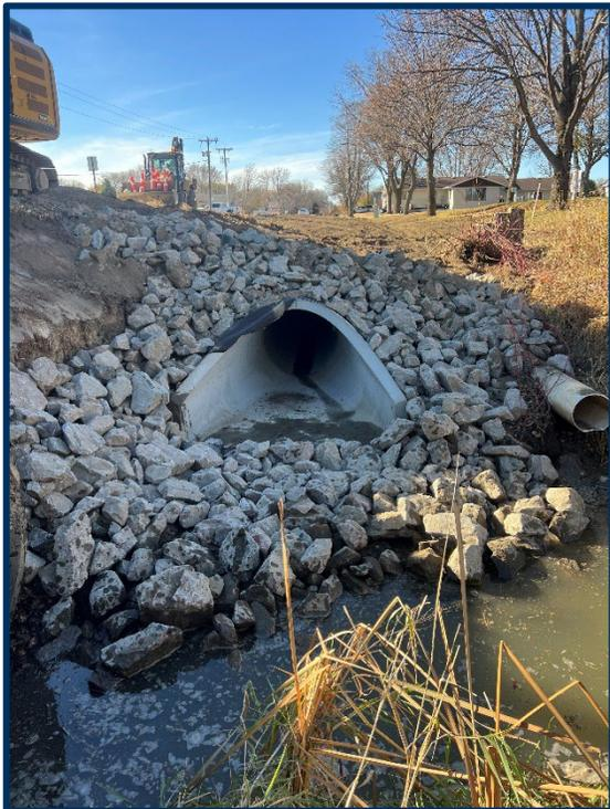
Installation of Class III Riprap around the 36" RCP apron at approx. STA 32+40, looking west.
