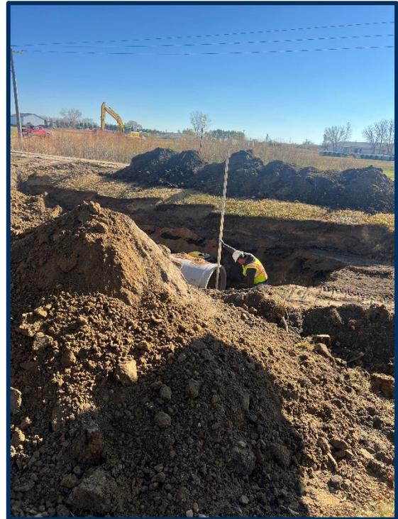
The Contractor performing invert elevation checks on installed RCP. Approx. STA 31+75, looking southeast.
