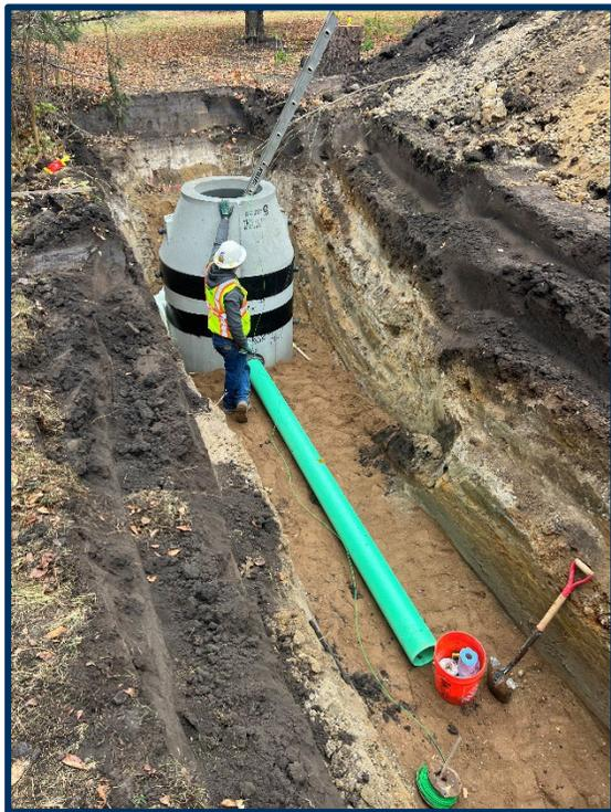
Installation of SMH #17 and sanitary sewer pipe using sand bedding material. Approx. STA 68+65, looking southeast.
