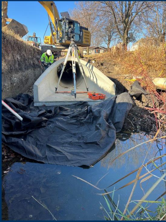
Installation of the 36" RCP apron and Type IV Geotextile Filter. Approx. STA 32+30, looking west.
