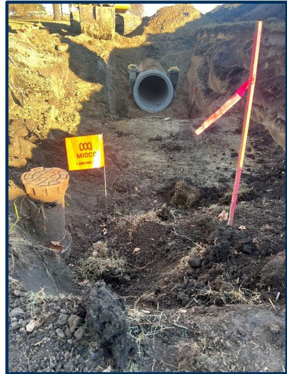
Existing 4" water valve near alignment of 36" RCP storm sewer. The pink lath represents the centerline of the 36" pipe to be installed. The orange flag represents the outside edge of the 4" water pipe. Approx. STA 30+55, looking east.
